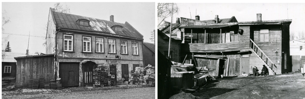
Illustration 1 and 2. Soviet period Supilinn waiting for demolition. On the left: 1992, Herne 6. Source: ERM Fk 2018:57, Duglas, H. On the right: 1992, Oa 3 courtyard house. Source: Tartu City Museum TM F 985:3, Duglas, H.
