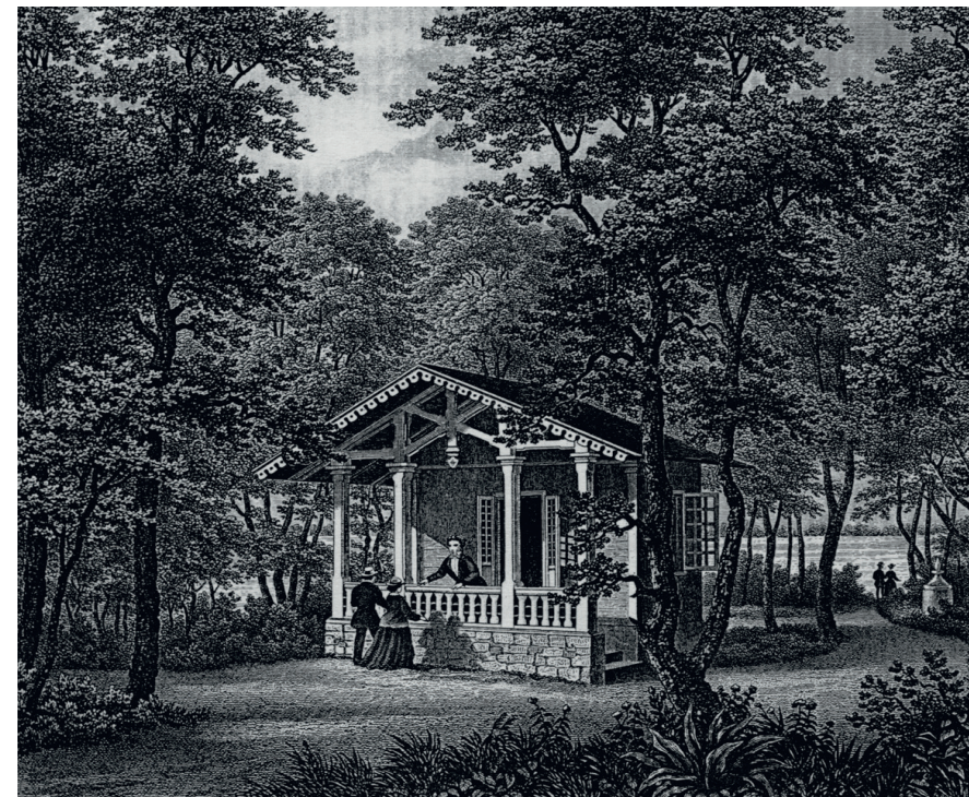
Ill. 11. Nn Schilleri majake, ehitatud 19. sajandi keskel. Kaugemal on näha Friedrich Schillerile püstitatud mälestussammas. Gravüür Wilhelm Siegfried Stavenhageni joonistuse järgi, 1866. TLÜ Akadeemiline Raamatukogu. / The so-called “little Schiller house”, built in the middle of the 19th century. In the distance, the monument erected in honour of Friedrich Schiller is visible. Engraving based on a drawing by Wilhelm Siegfried Stavenhagen, 1866. Academic Library of Tallinn University.
